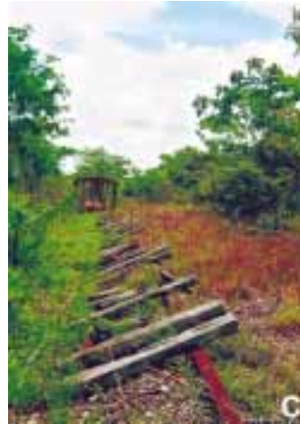
Picture 'C' shows a railway line. Clearance is complicated by the presence of wrecked carriages and by the fact that the line has been turned upside down, then booby-trapped.
