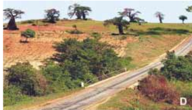
Picture 'D' shows an open hillside in Africa. The heavily overgrown road bridge has been mined and the suspect area extends among the baobab trees where goats are allowed to graze.
